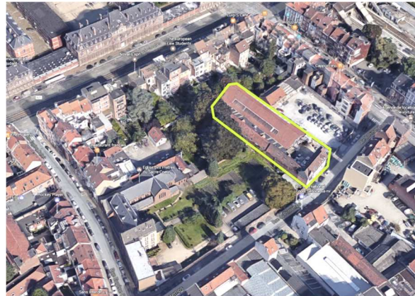
Figure 12 : View of the land lot in google map, earlier building in yellow
