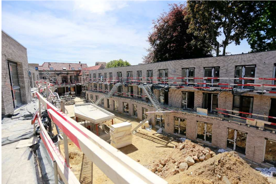
Figure 37 : View on the inside yard from the AI unit
