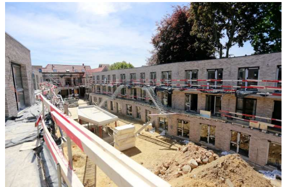
Figure 3 : View from unit A1 balcony towards interior yard, during construction work
