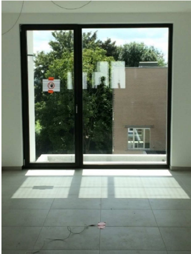
Figure 20 : Internal view in the living room unit B, effect of the shade screen
