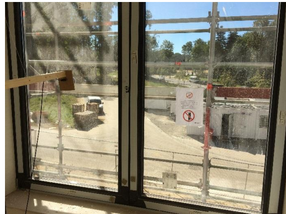
Figure 20 : View of the scaffold, Unit BI
