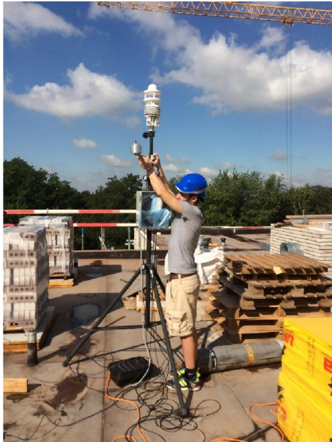
Figure 28 : Weather station on the roof
