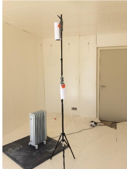
Figure 27 : Electric radiator in the insulated unit (AI)
