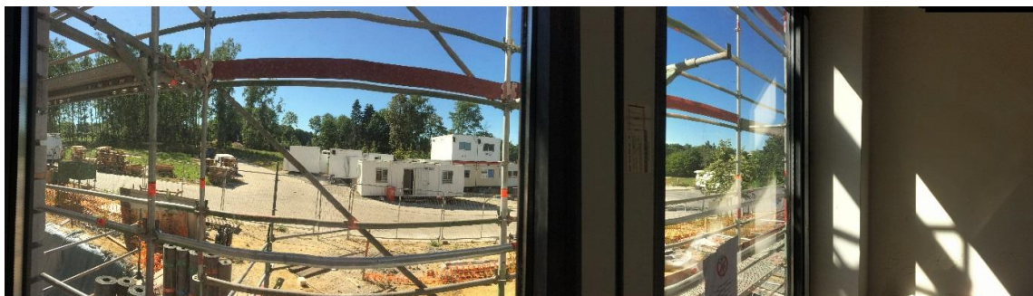
Figure 30: Panoramic view toward the window of unit AU
