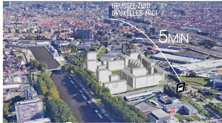
Figure 2: 3D view of the location of the Citydox complex (source : citydox.be)
